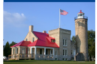
Mackinac Point Lighthouse
